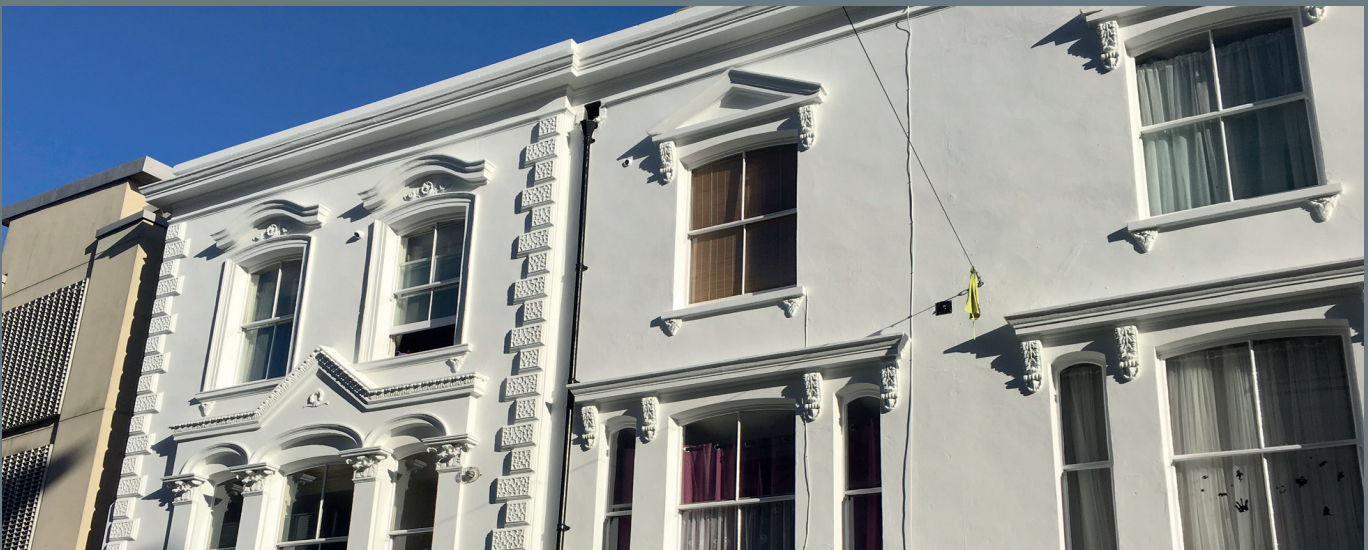
Reinstatement of 1st & 2nd Floors with Stucco Detailing
